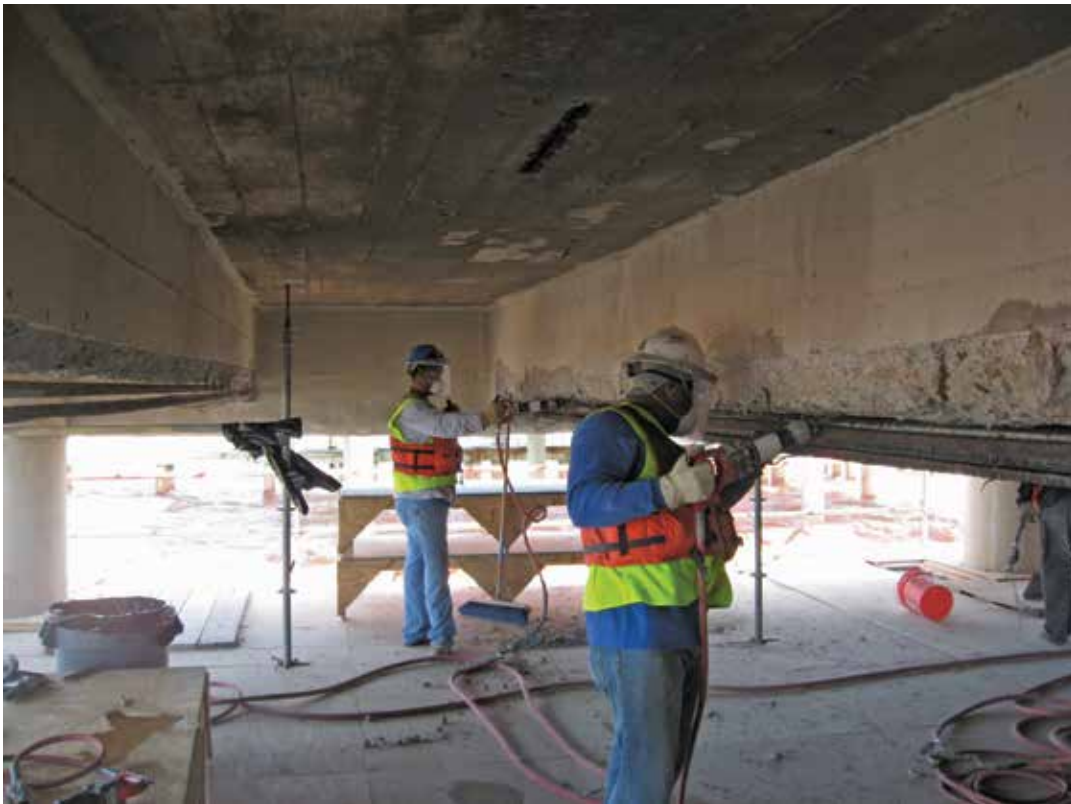
Fig. 2: Surface preparation of deck support beams
