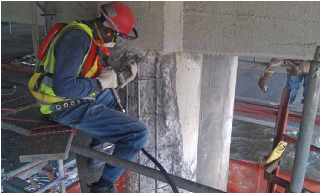
Fig. 3: Surface preparation of pier columns
